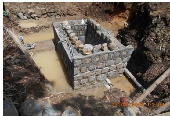
Spring Catchment construction in Moh
