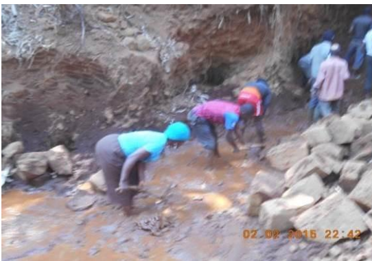
Spring excavation in Bamngam
