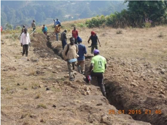
Pipeline excavation in Kungi
