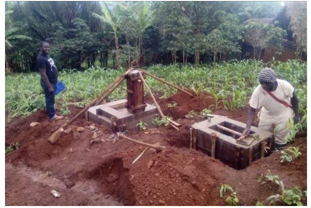
Construction of standpipe and meter chamber
