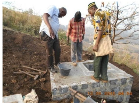
Coordinator inspects completed catchment in Bamngam
